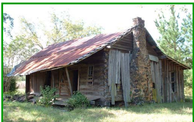
The camera is looking northwest in this photo. The original chimney is on the east side of the house. The kitchen area was added to the back of the house.
